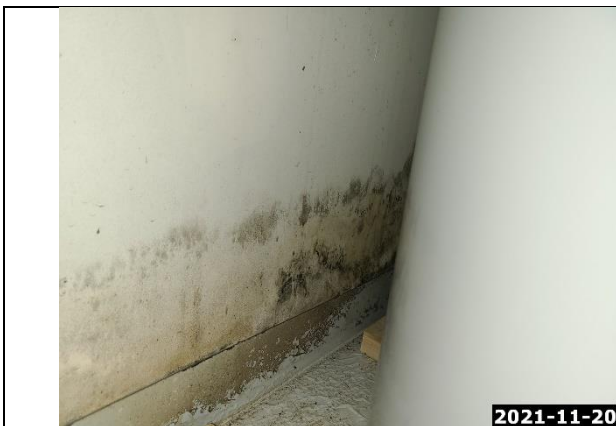
Laundry Room / AC Closet
