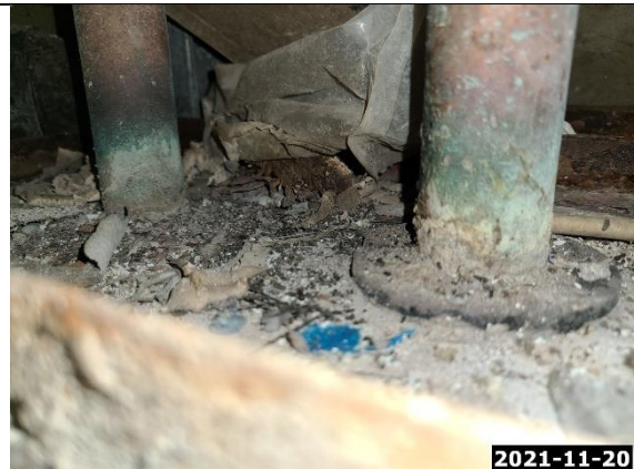
Laundry Room / AC Closet
