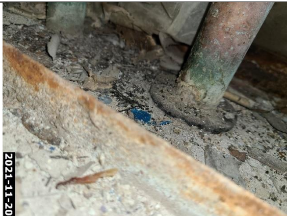
Laundry Room / AC Closet
