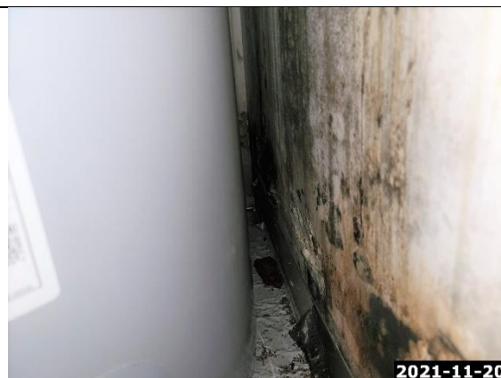
Laundry Room / AC Closet
