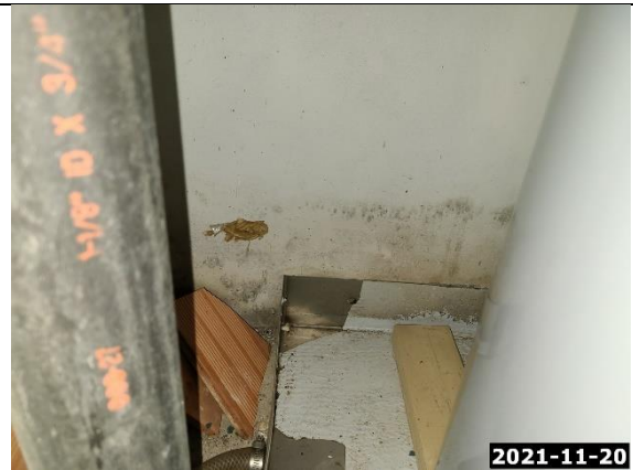
Laundry Room / AC Closet
