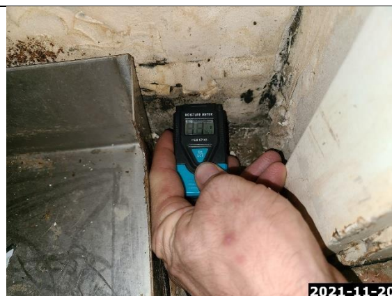
Laundry Room / AC Closet
