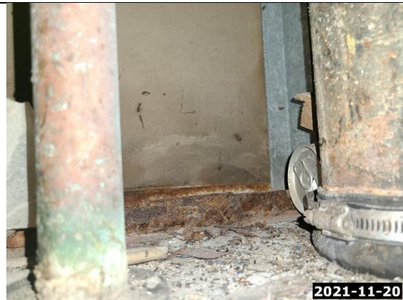
Laundry Room / AC Closet
