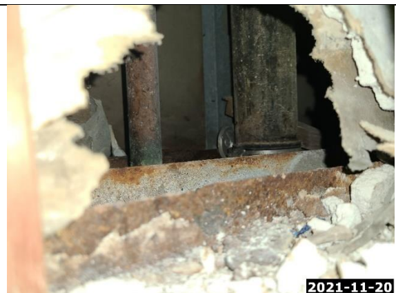
Laundry Room / AC Closet
