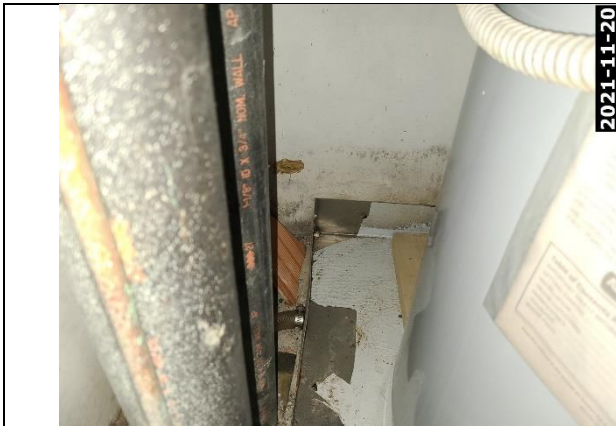
Laundry Room / AC Closet
