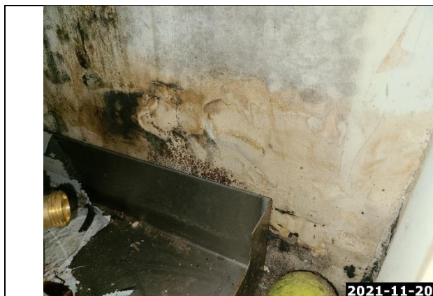
Laundry Room / AC Closet
