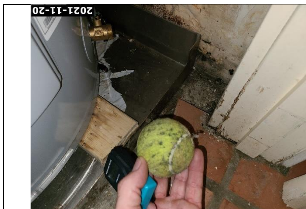
Laundry Room / AC Closet
