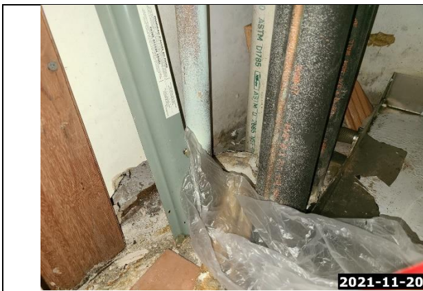
Laundry Room / AC Closet
