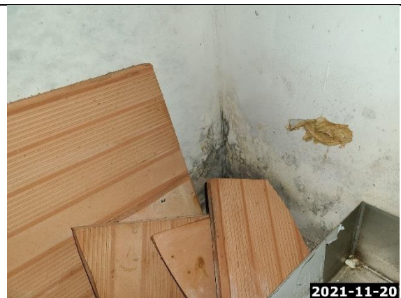
Laundry Room / AC Closet
