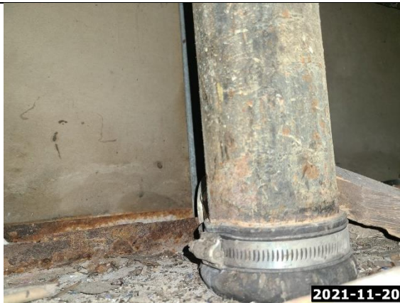
Laundry Room / AC Closet
